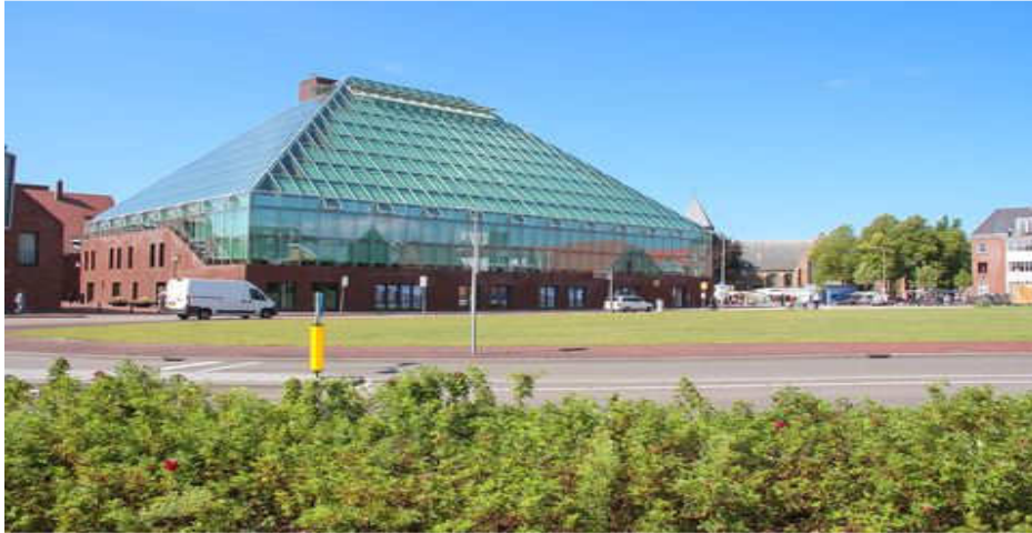
Fig. 38. Spijkenisse Public Library Foundation, Spijkenisse, Netherlands
