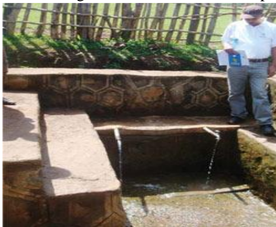
Figure 1.2: A protected spring Source: WaterAid, Ethiopia
