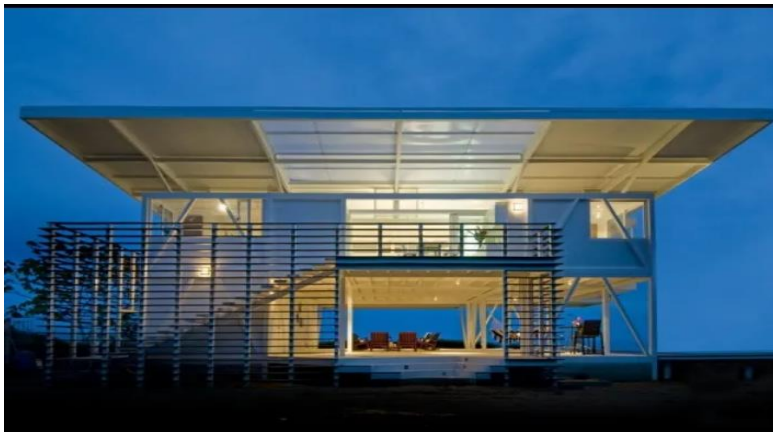
Fig.5.9: The White Steel Villa in Costa Rica
